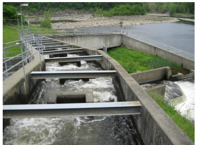
This photo shows a close-up of the Spillway Ladder—an Ice Harbor type pool-and-weir fishway. When the amount of water spilling over the dam is low, few fish come up this far to use this fishway. Fish that use this ladder still must pass through the Gatehouse ladder to get out of the canal and into the headpond. (Both photos courtesy of Ken Sprankle, USFWS.)
