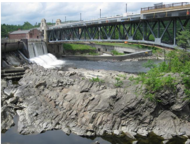
Last week, we ran a photo of the Cabot Station Powerhouse at Turners Falls at the downstream end of the power canal. Here we show you the Spillway ladder at the upstream end of the canal. Fish that overshoot the Cabot Ladder down by the powerhouse come up to the dam and can use this fishway, seen beyond the Rt. 2 bridge.
